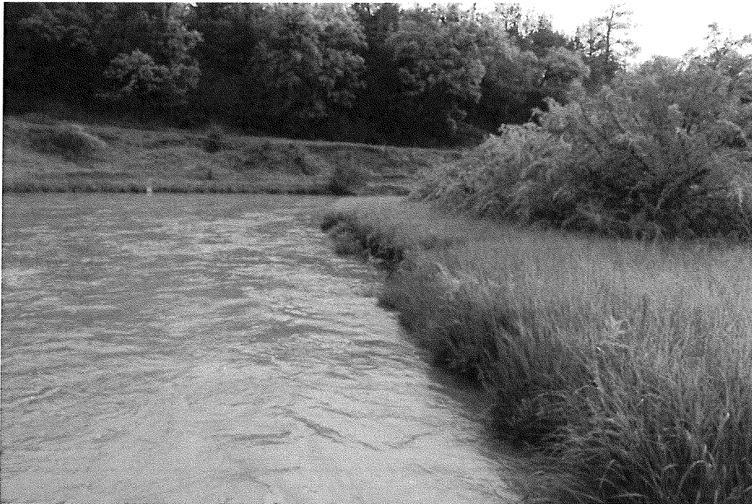
Photo 7 - Opposite bank with heavy grass growth. Note cut cedars.
